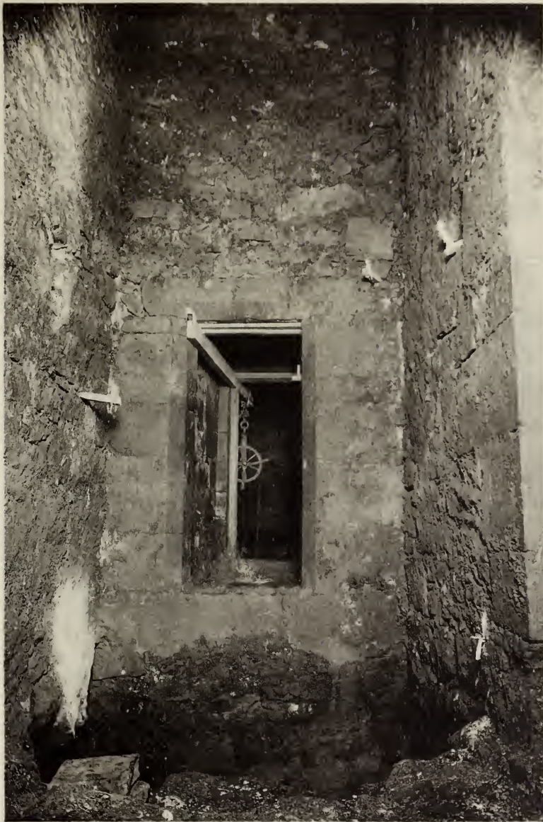
(FIG. 12) VIEW OF SOUTH SIDE OF ENTRANCE HALL, SHOWING LATER DOORWAY AND SUNK PIT
